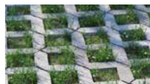
GRASS BLOCK PAVERS interlocking concrete paving cells filled with grass seed or turf
